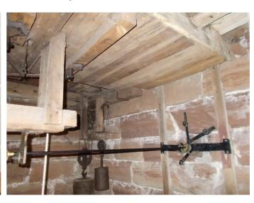
June 2017 automatic winding installed: extra framework clamped (not bolted) to existing frame, new weights & pulleys, battery backup attached to cupboard
